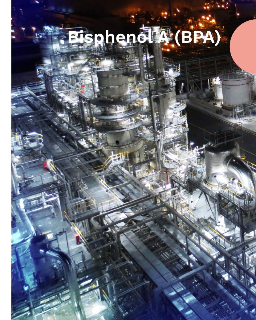
The Badger Bisphenol A (BPA) technology converts commercial grade phenol and acetone into high-purity BPA suitable for polycarbonate, epoxy resin, and other chemical applications.
